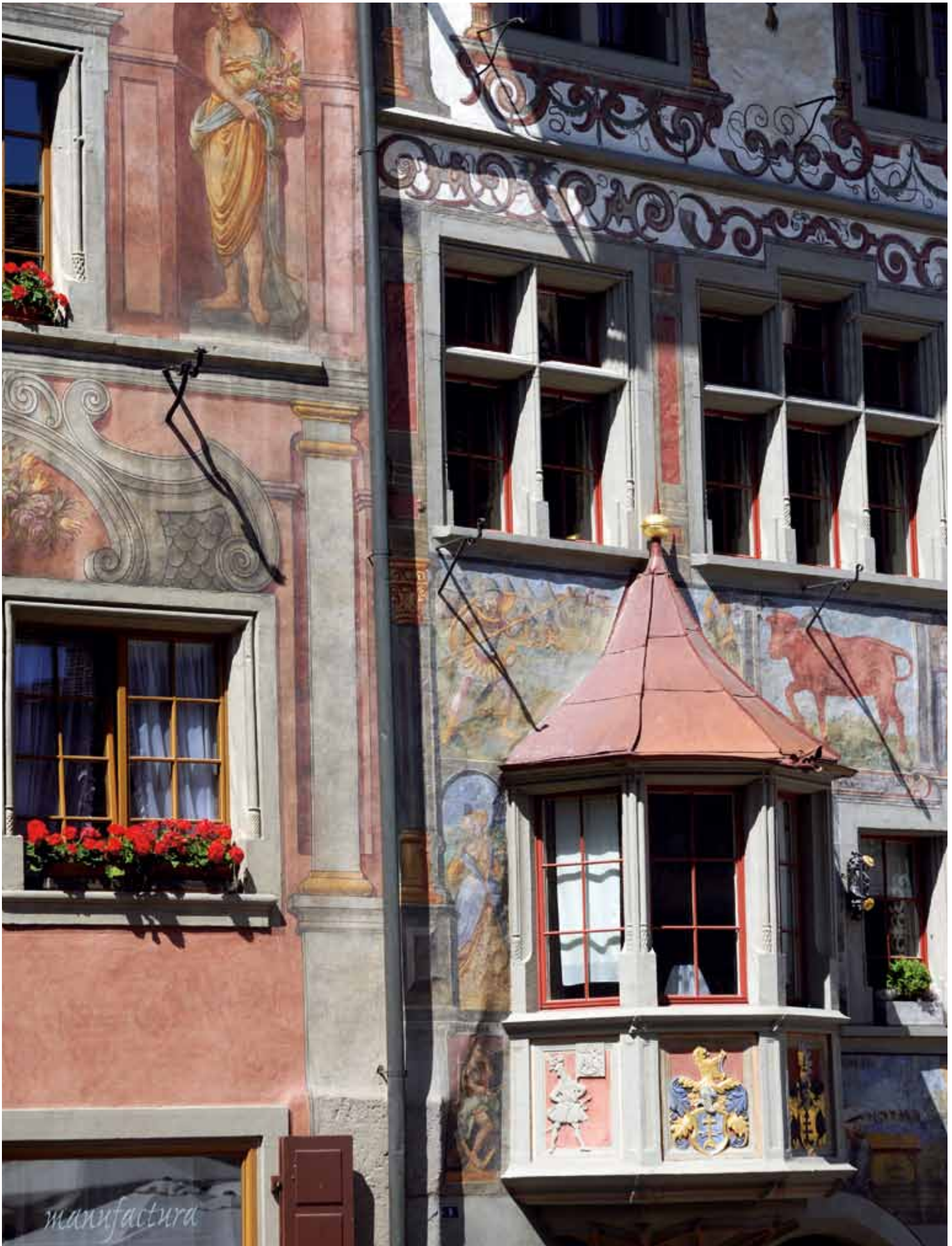
Residential and commercial building, Stein am Rhein (CH); original coating from 1900
